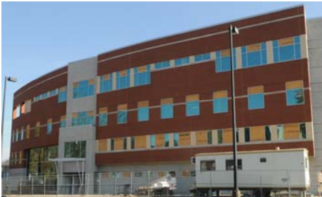
The new ChER building nearing completion.
